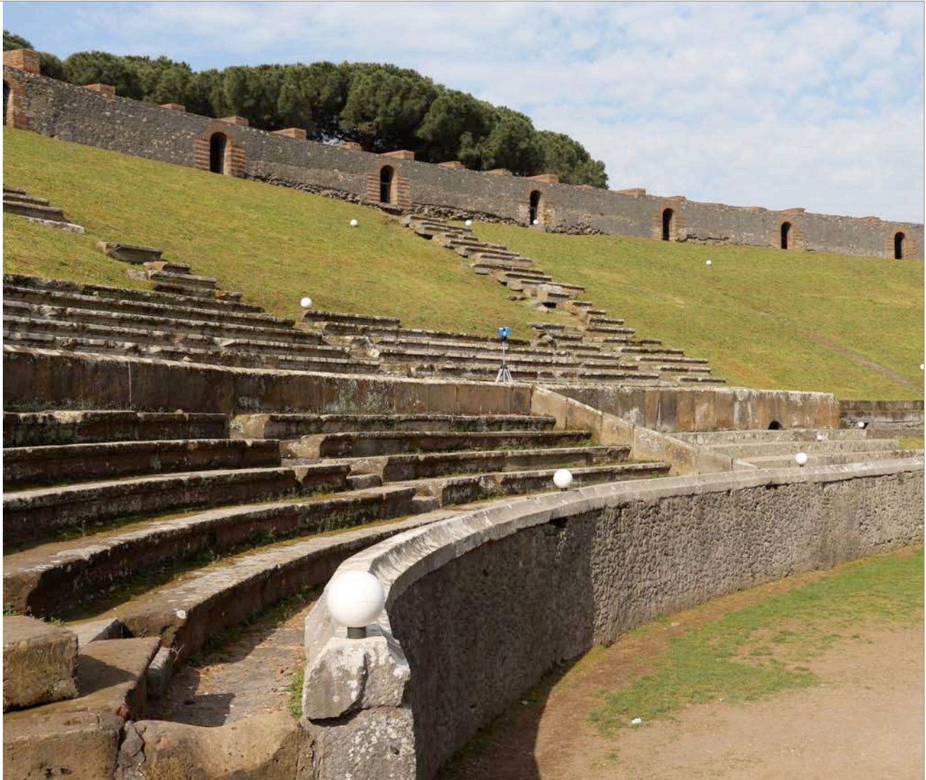
Fig. 26: Pompeii, Amphitheatre. A instant view of the cavea during the capturing laser data. In the scenario there are many white spherical targets.
