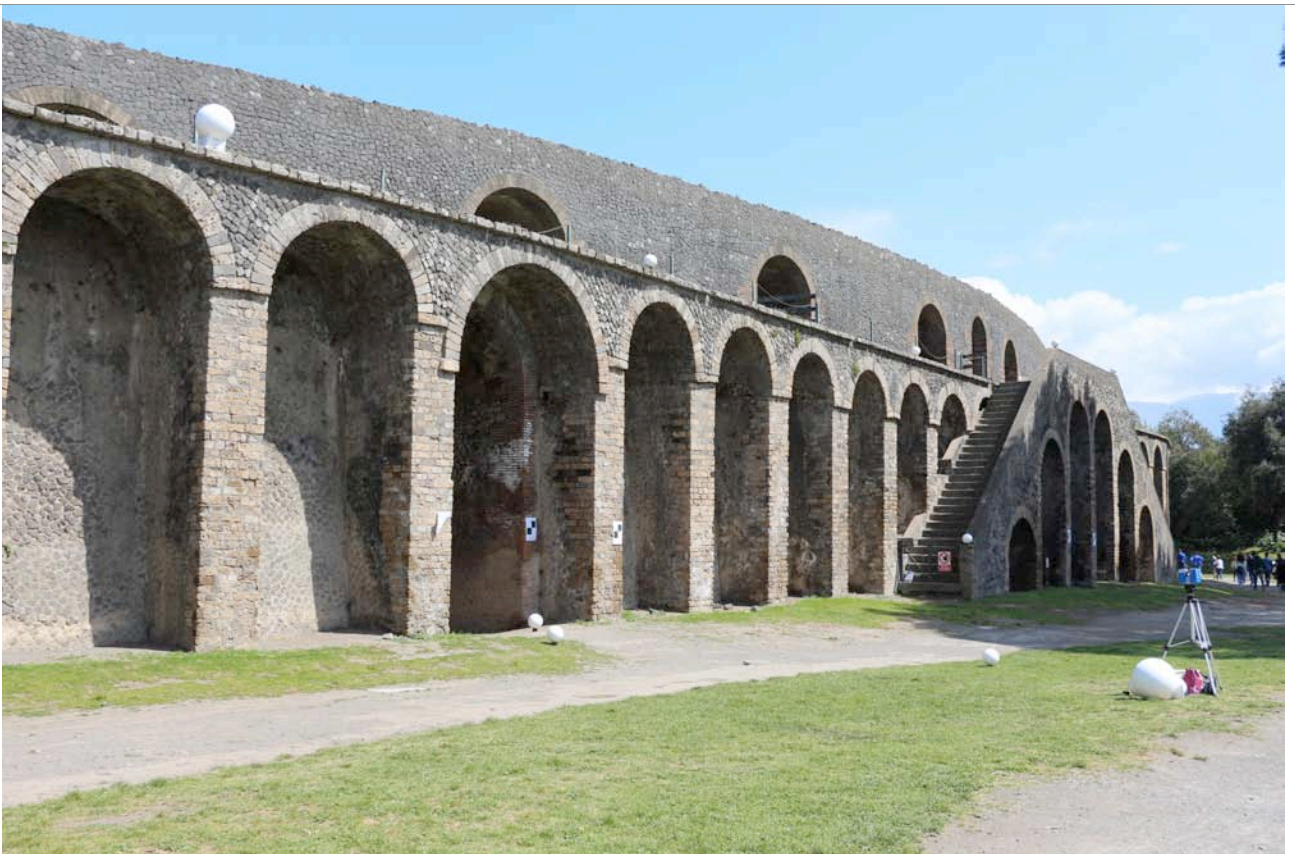
Fig. 28: Pompeii, Amphitheatre. A instant view of the perimetrical arches during the capturing laser data. In the scenario there are many white spherical targets.
